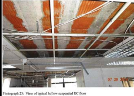
Photograph 23: View of typical hollow suspended RC floor
