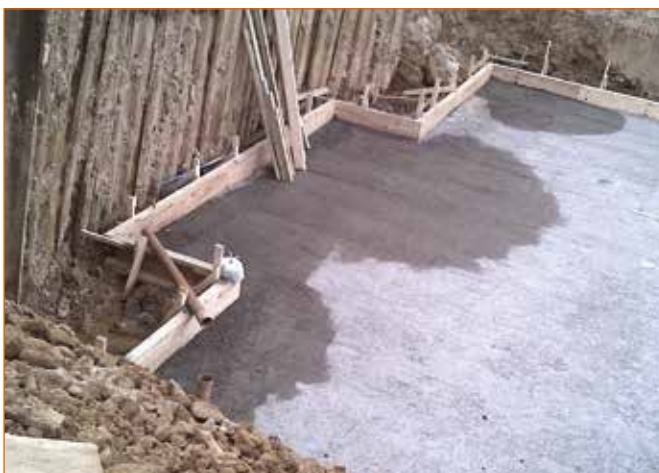
Image 1: Basement being constructed below ground
