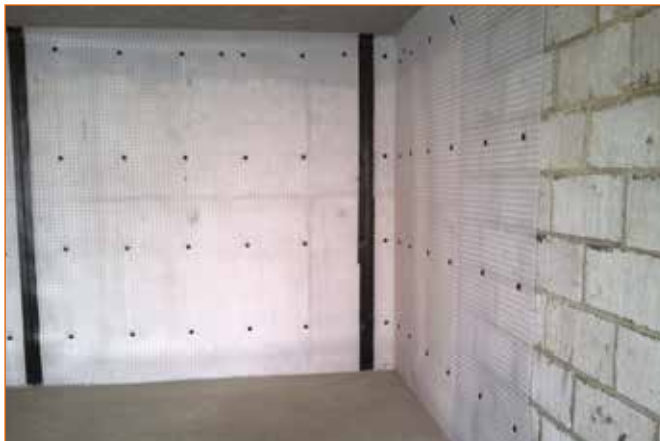
Image 2: Example of internal damp proof membrane
