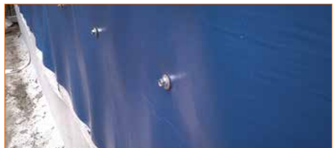
Image 3: Example of external damp proof membrane
