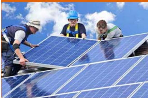
Image 1: Installing panels generally results in an increase in dead load of around 15%.
